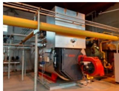
Obr. 7: Parní kotel UNIVERSAL UL-SX-IE 8000x18
