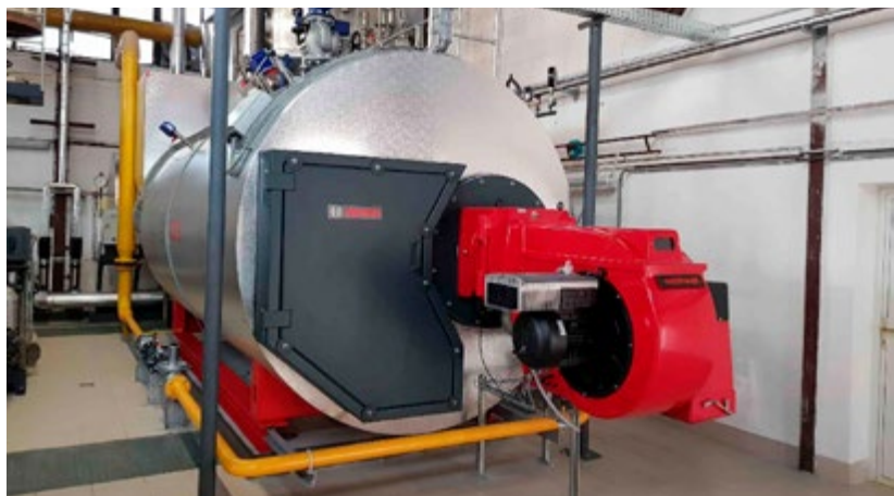
Obr. 5: Parní kotel UNIVERSAL UL-S-IE 7000x13
