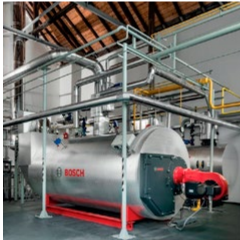
Obr. 2: Parní kotel UNIVERSAL UL-S-IE 4000x10
